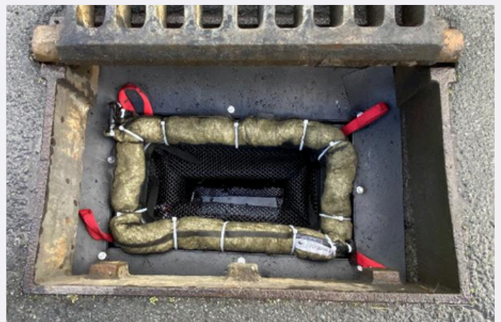
LavaSorb™ boom set up with LittaTrap™ to ensure it absorbs oils and oil-based liquids in the stormwater.
